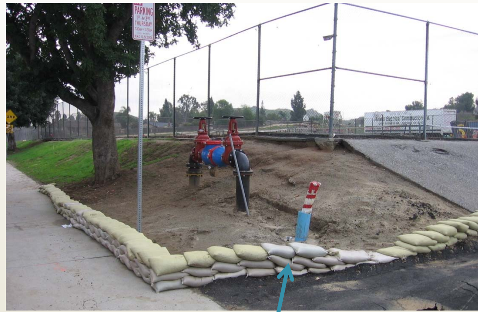
The ends of the bags should overlap.
