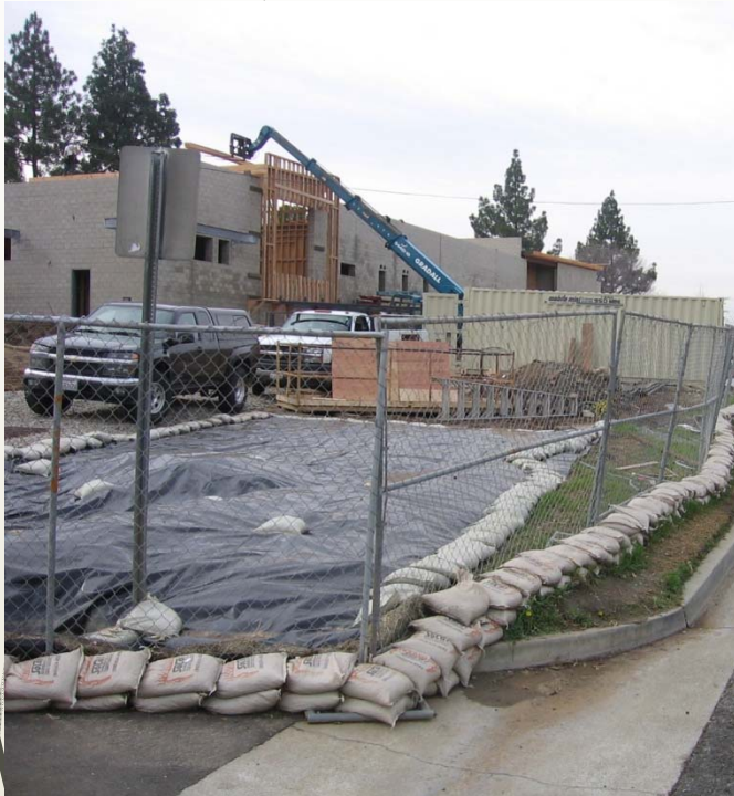
Multi-layer gravel bag linear barrier.
