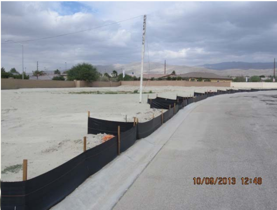
Silt fence linear barriers. Stakes are on the downgrade side.
