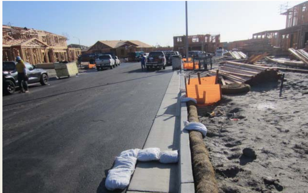
Gravel bag check dams in curb flow lines
