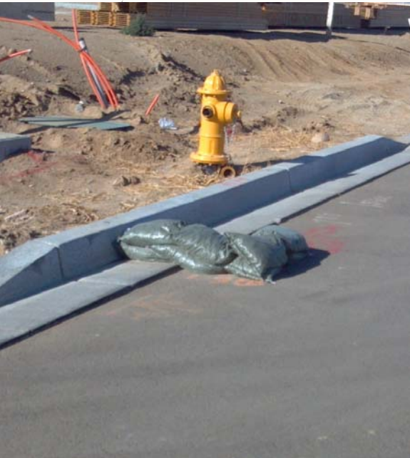
Gravel bag check dams in curb flow lines
